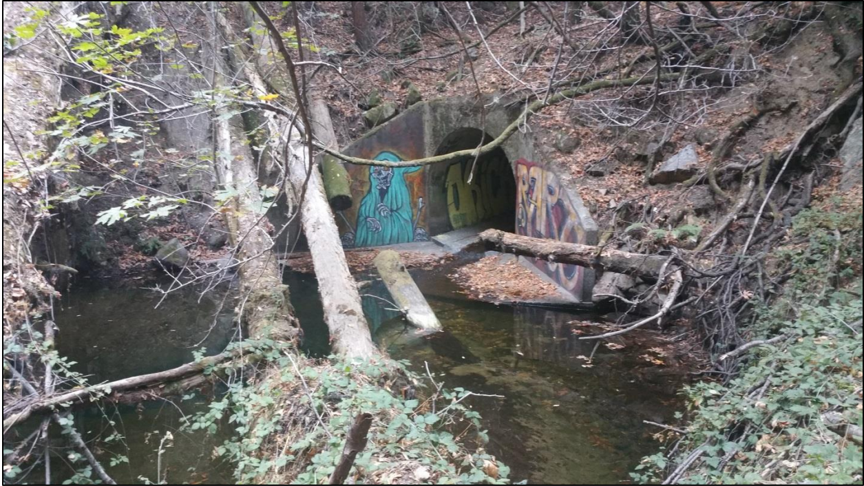
Figure 24: Hwy 17 Aldercroft Culvert: Northbound, east side on September 2016.
