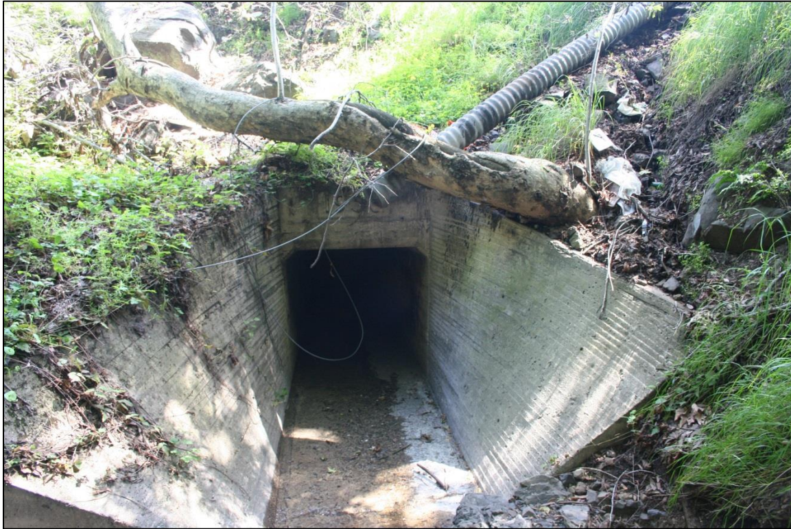
Figure 22: Ravine Culvert, southbound, west side.
