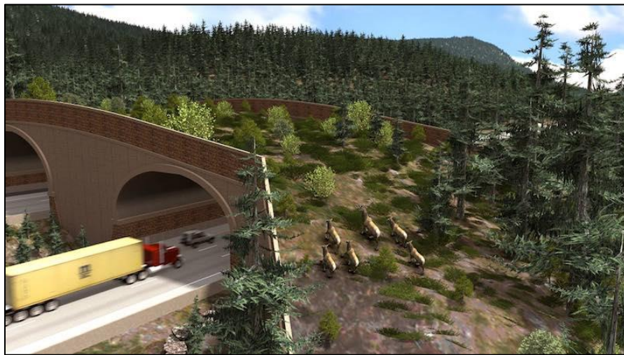
Figure 39: I-90 Landscaped wildlife bridge-Washington State Transportation Dept.
