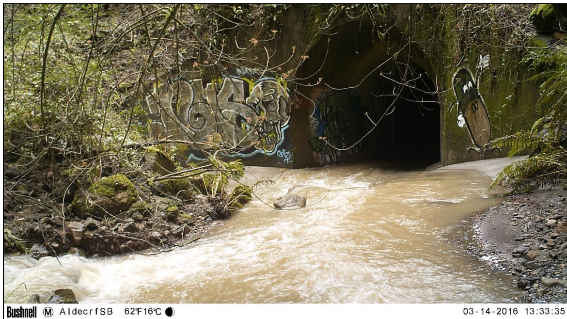
Figure 23: Hwy 17 Aldercroft Culvert: Southbound, west side on March 2016.
