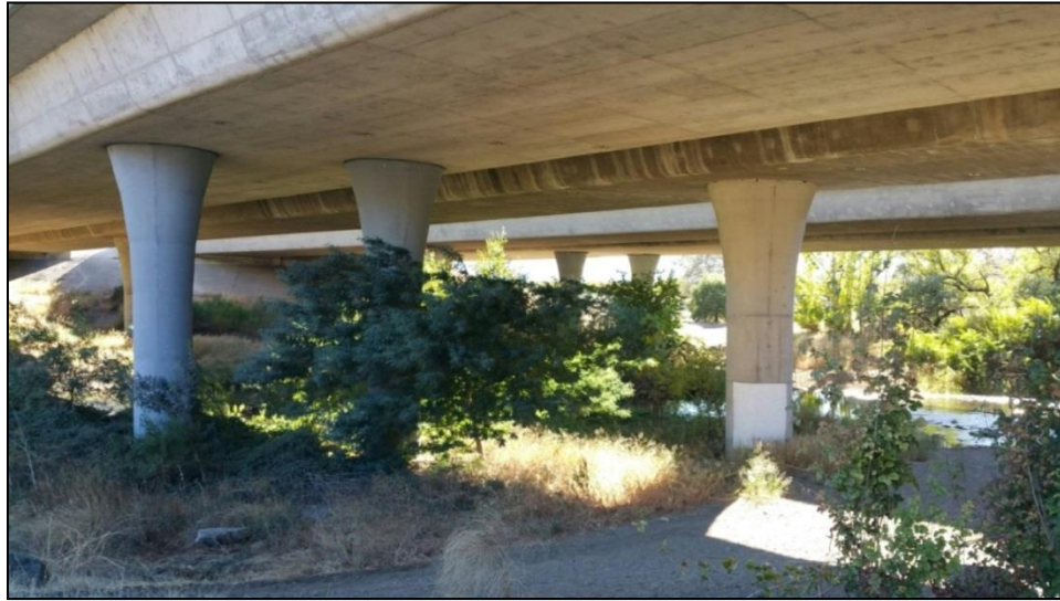
Figure 49: Highway 101 Coyote Creek Underpass.
