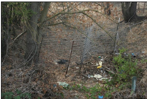
Figure 16: Fencing on north side of Palm Bridge.
