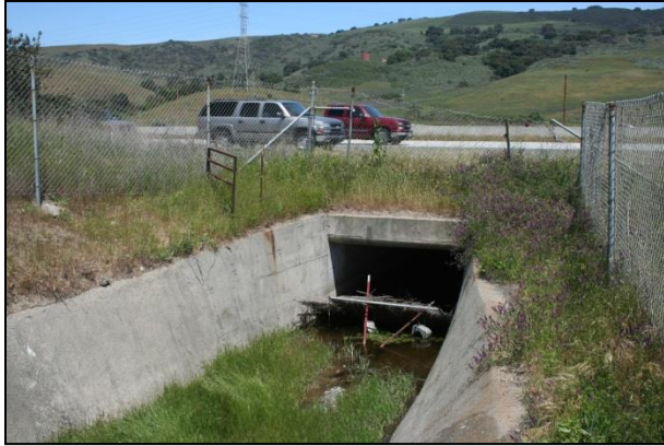
Figure 18: Hwy 101 Culvert 23 blocked by fence. Figure 19: Hwy 101 Culvert 21 full of debris.
