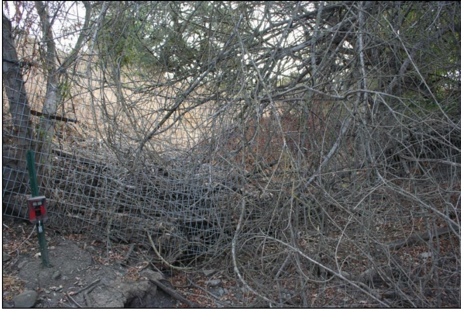
Figure 33: Exclusionary Fencing on south side of the Bailey bridge in Fisher Creek.
