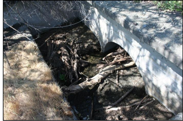
Figure 18: Hwy 101 Culvert 23 blocked by fence. Figure 19: Hwy 101 Culvert 21 full of debris.
