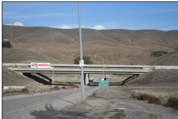
Figure 42: Highway 101 Golf Course Drive Underpass.
