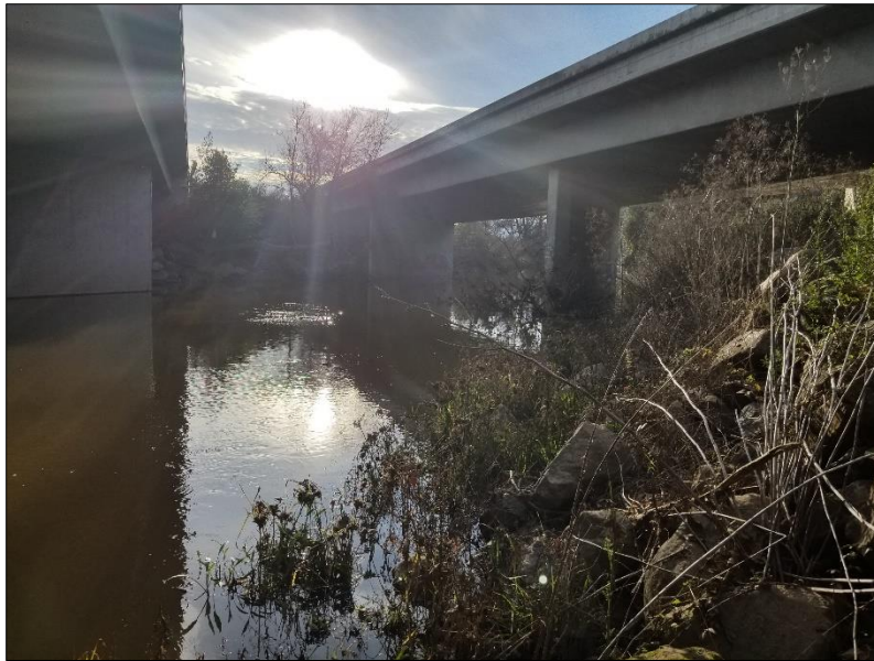
Figure 15. Pacheco Creek bridge flooded during February 2019.
