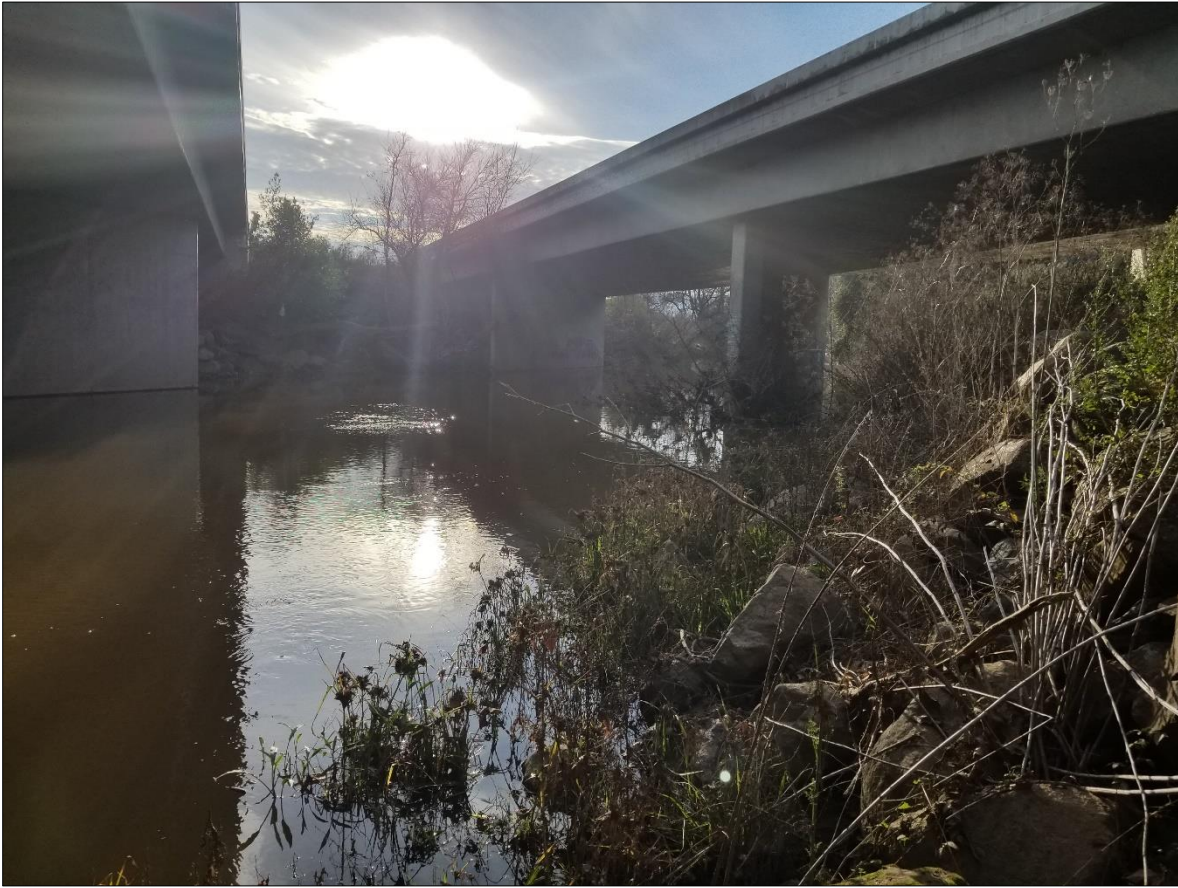
Figure 21. The east side of the Pacheco Creek bridge.
