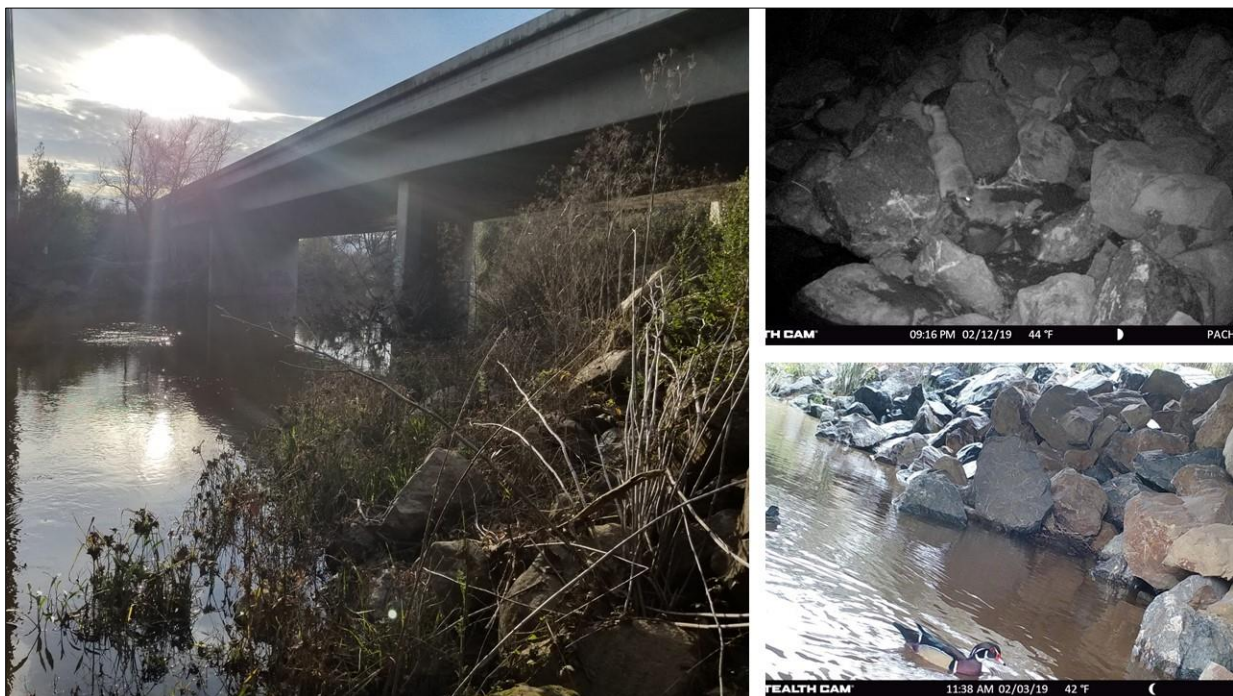
Figure 18. Pacheco Creek bridge in February 2019 and camera data.
