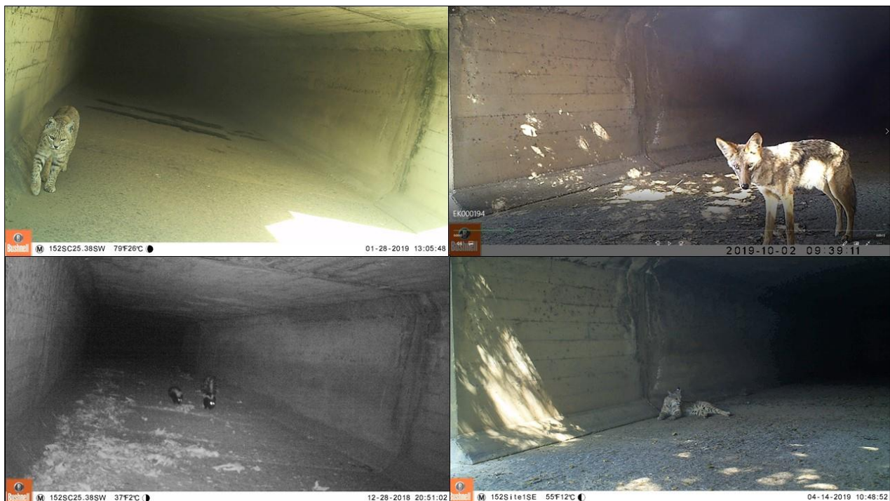
Figure 5. Multiple species use of the Elephant Head creek culvert.
