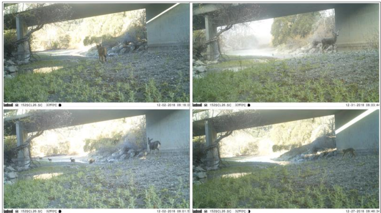
Figure 7. Multiple species use of the Pacheco Creek bridge middle east section.
