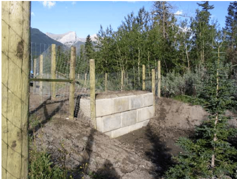
Escape ramp (jump-out) for wildlife trapped inside highway right-of-way. Photo by Tony Clevenger.
