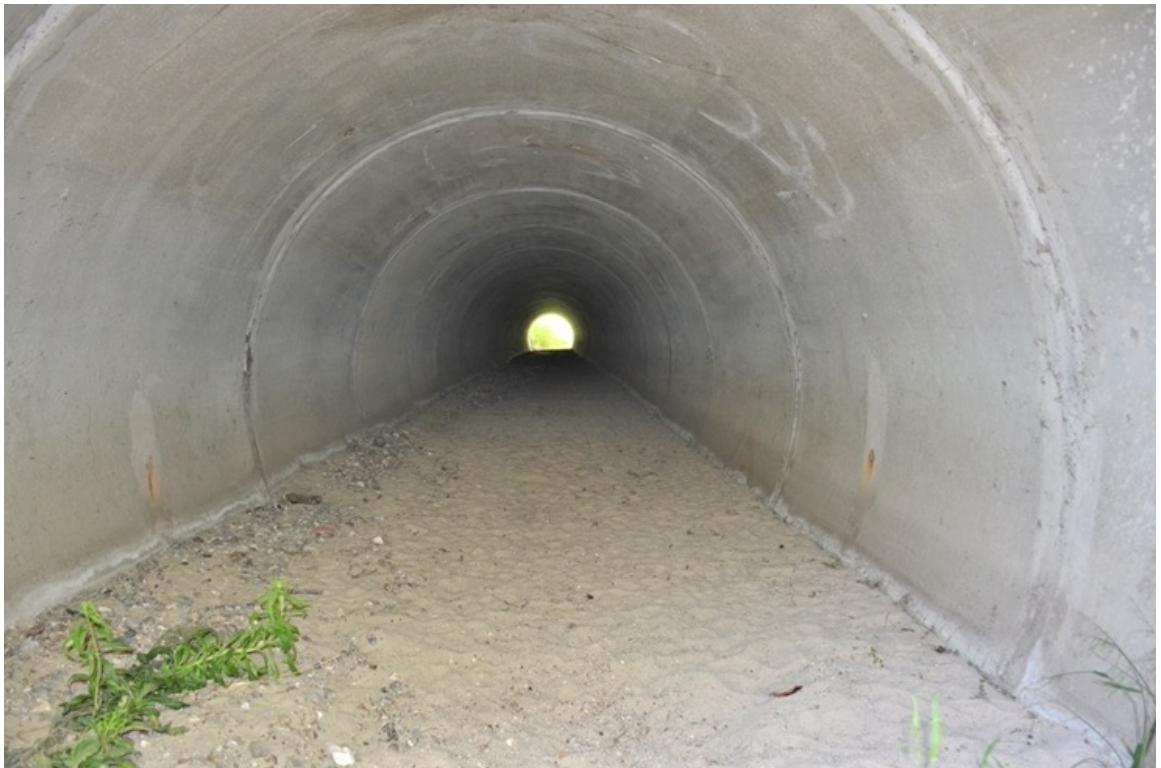
US 101 Site 20A. Within round culvert. Photo faces east.
