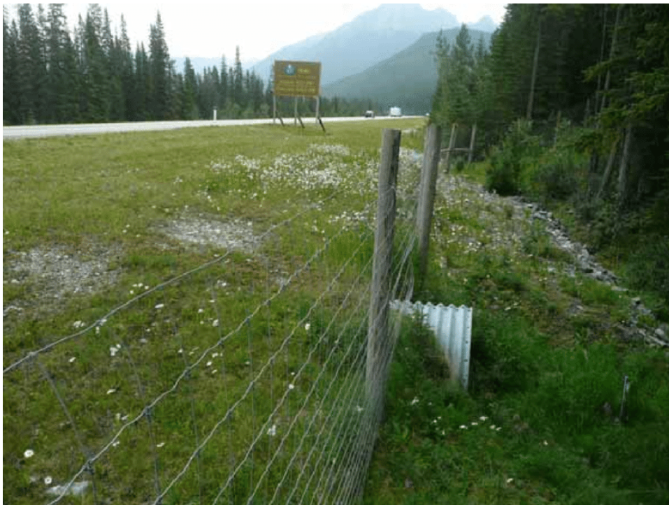
Wildlife exclusion fencing and culvert undercrossing. Photo by Tony Clevenger.
