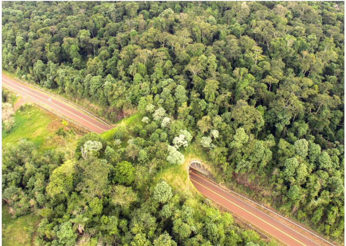
Example of a wildlife overpass near Iguazu, Argentina. Photo by Limba-Film Drone Project.
