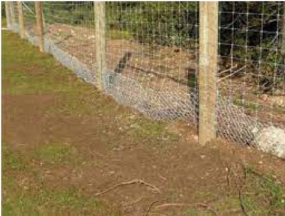
Wildlife exclusion fence with buried apron. Photo by Tony Clevenger.
