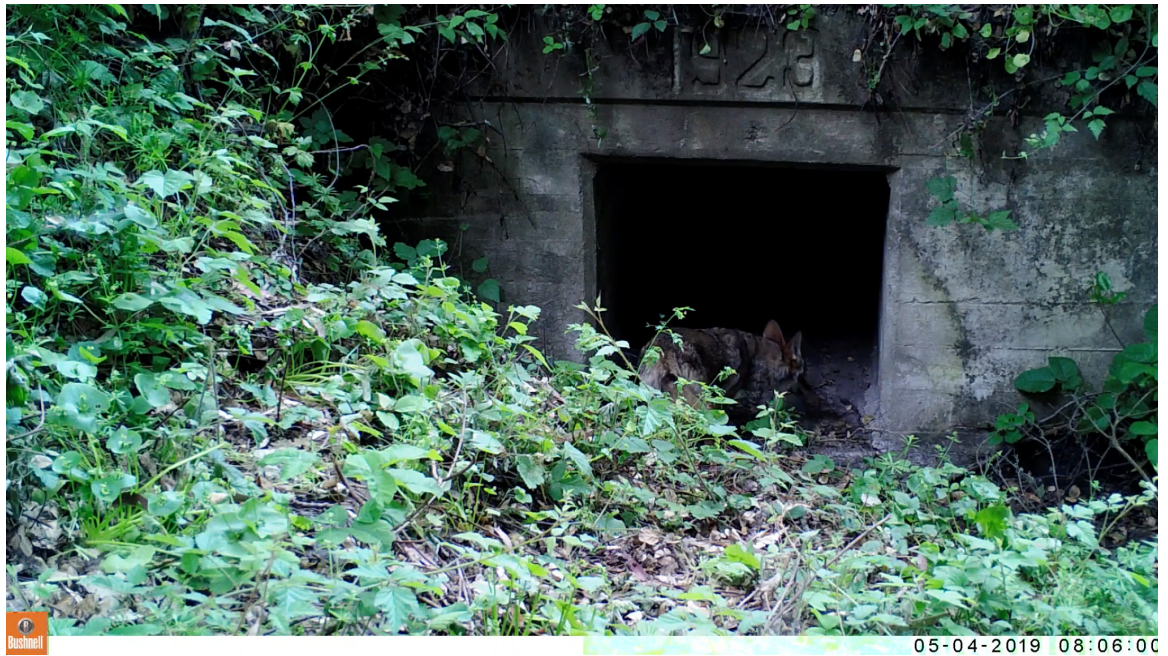
Coyote traveling through the SR 129 Site 3 culvert on May 4, 2019.
