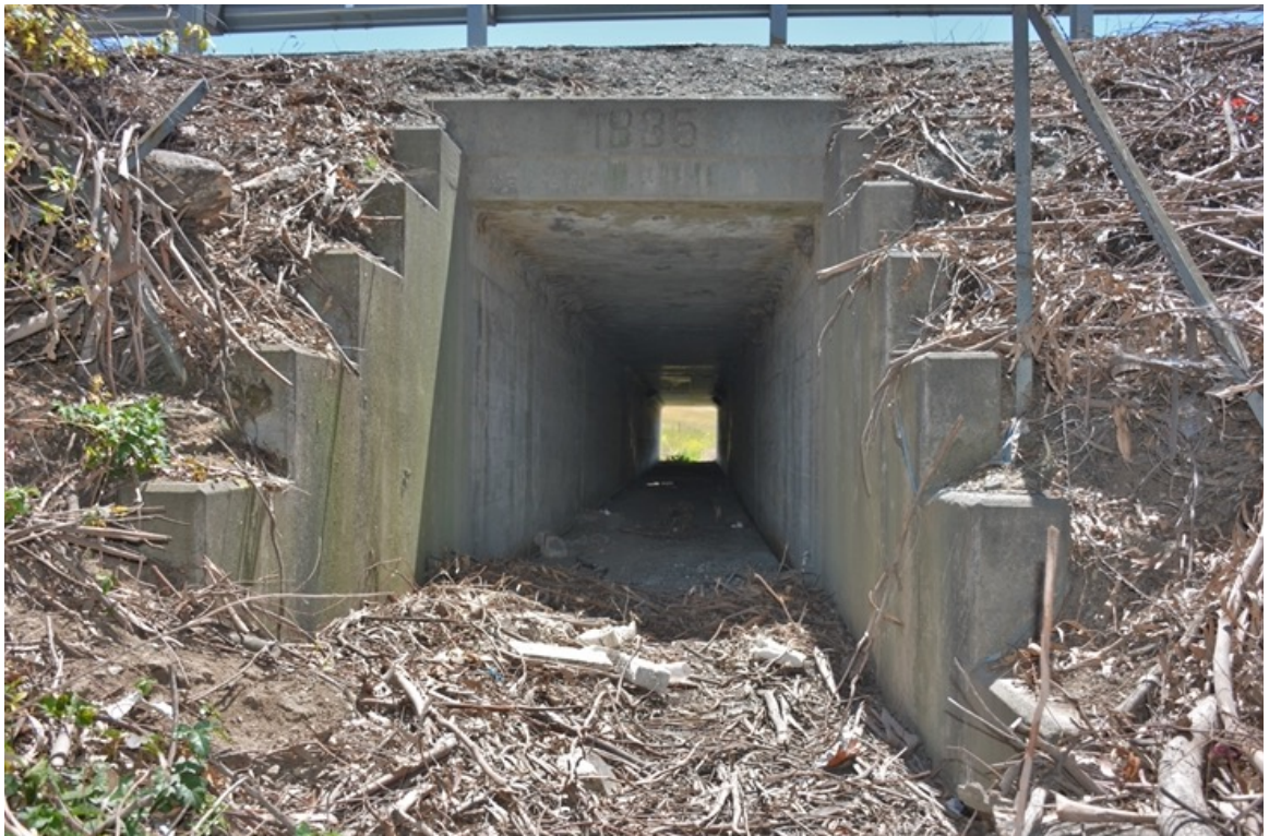
SR 156 Site 1. Northeastern opening. Photo faces southwest.
