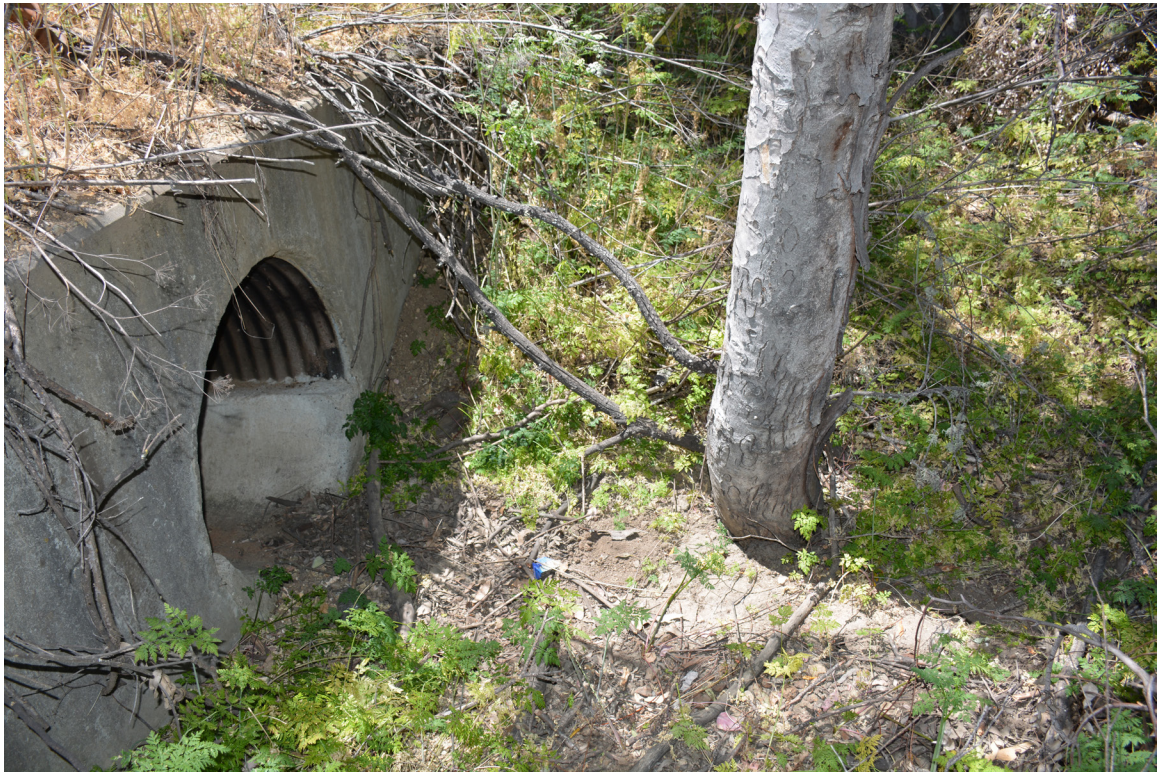
SR 156 Site 2. Northern opening.
