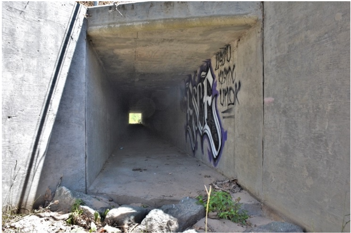
US 101 Site 16. Northeastern opening.
