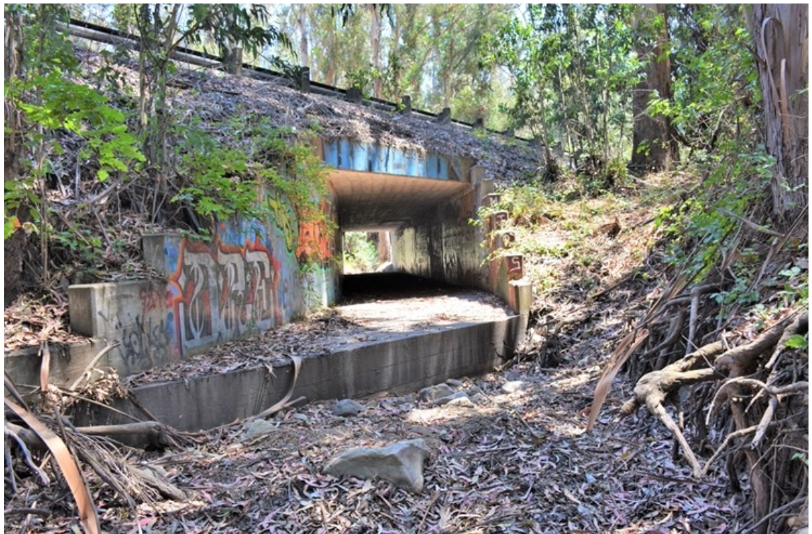
US 101 Site 9. Southern opening (in highway median).
