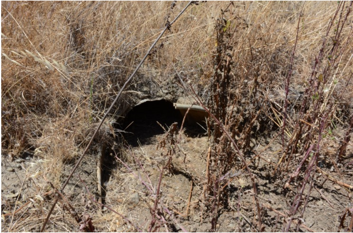
US 101 Site 6. Culvert to the west under Searle Road.
