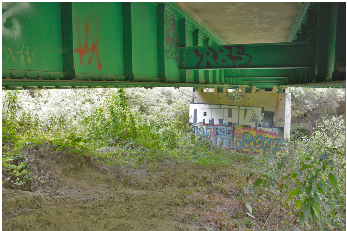
SR Site 5 Pajaro River Bridge. Western section. Photo faces east.
