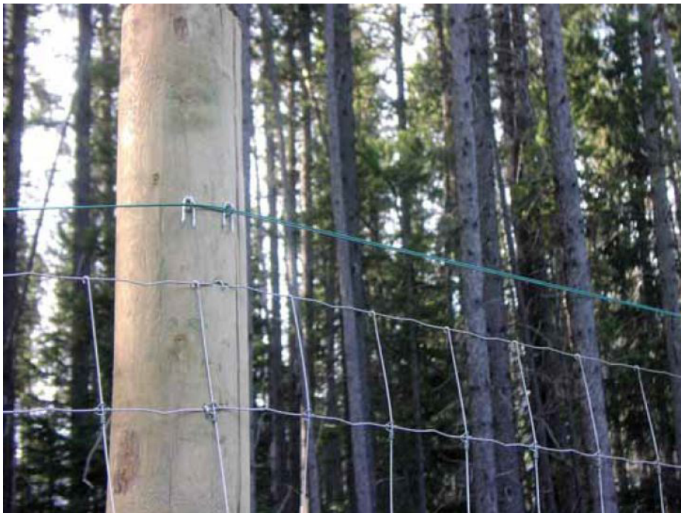
High tensile cable designed to break fall of trees onto fence material. Photo by Tony Clevenger.
