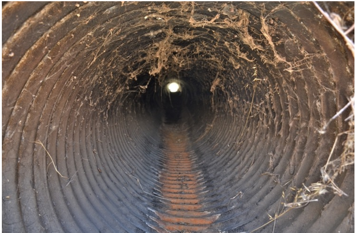
US 101 Site 6. Western opening close-up. Photo faces east.
