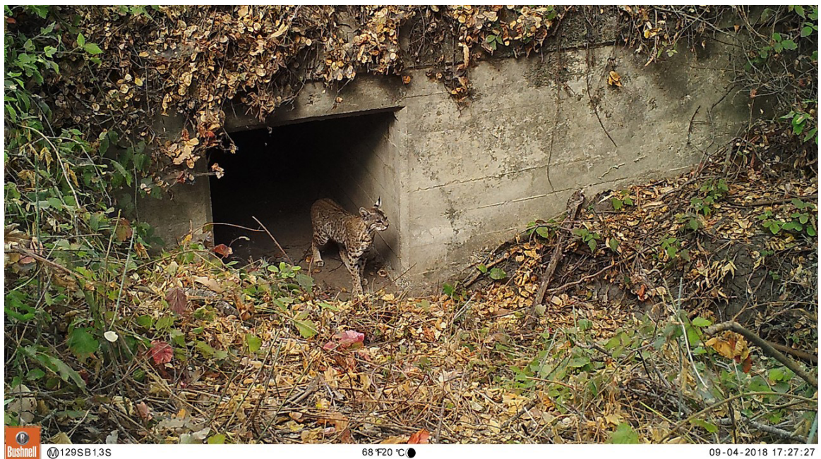
Bobcat traveling through the SR 129 Site 3 culvert on September 4, 2018.
