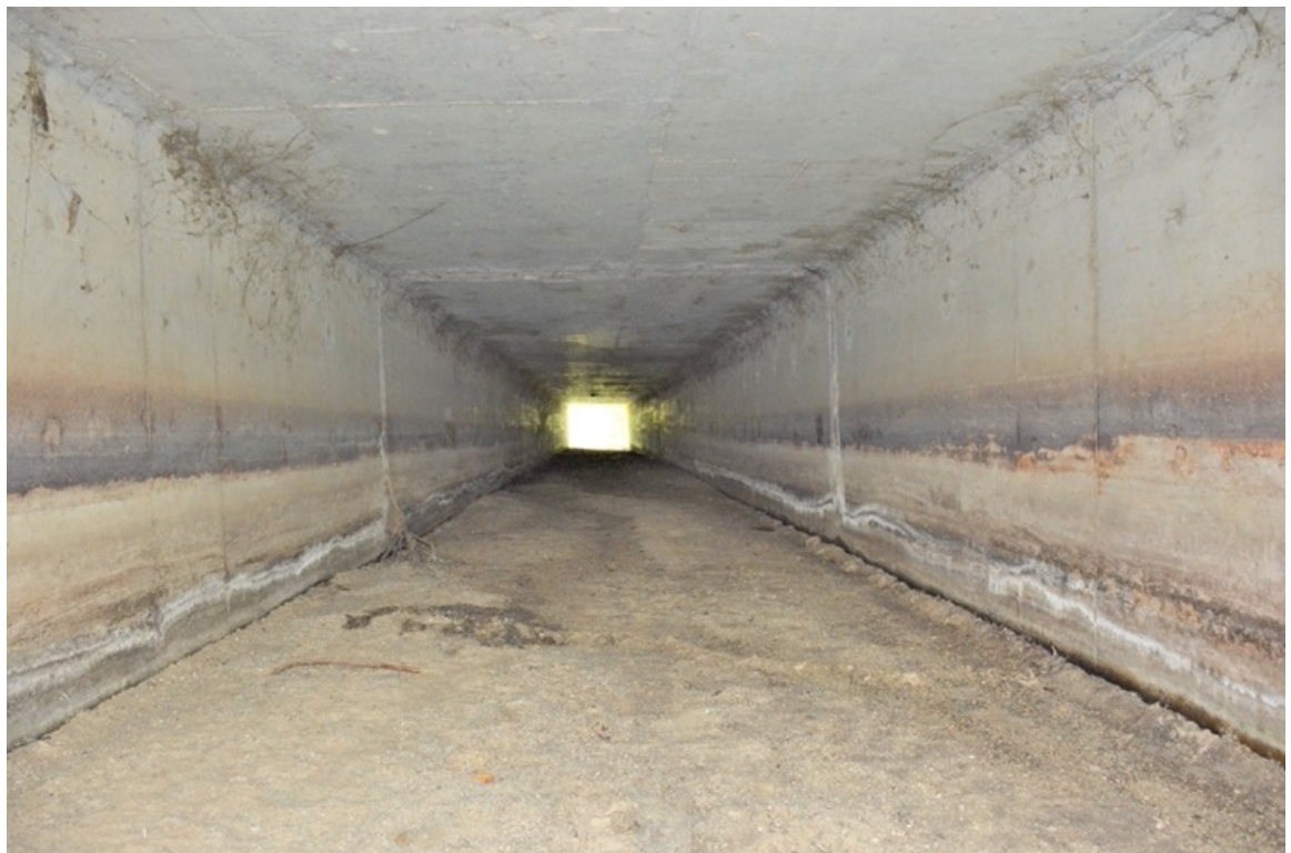
US 101 Site 20B. Within western opening facing east.
