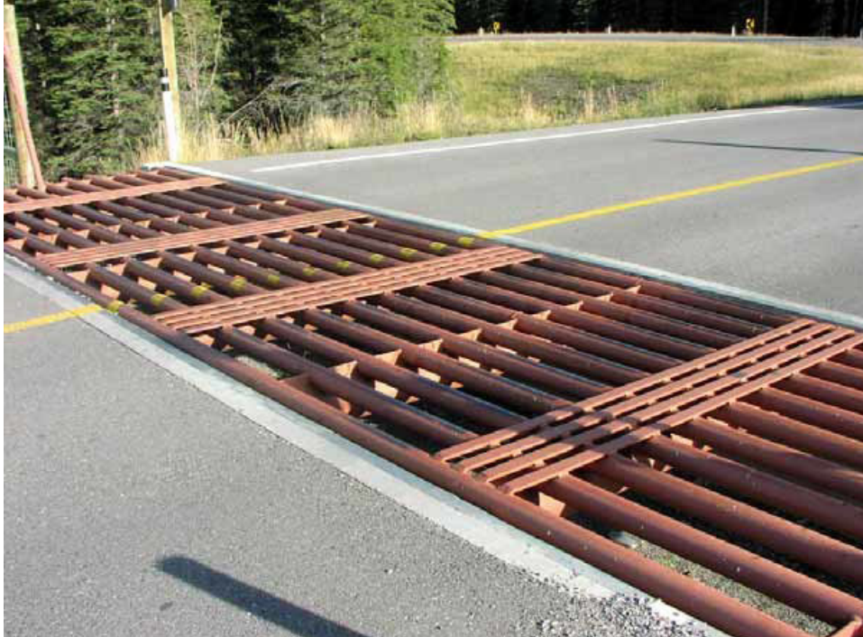
Cattle guard (Texas gate) in road. Photo by Tony Clevenger.
