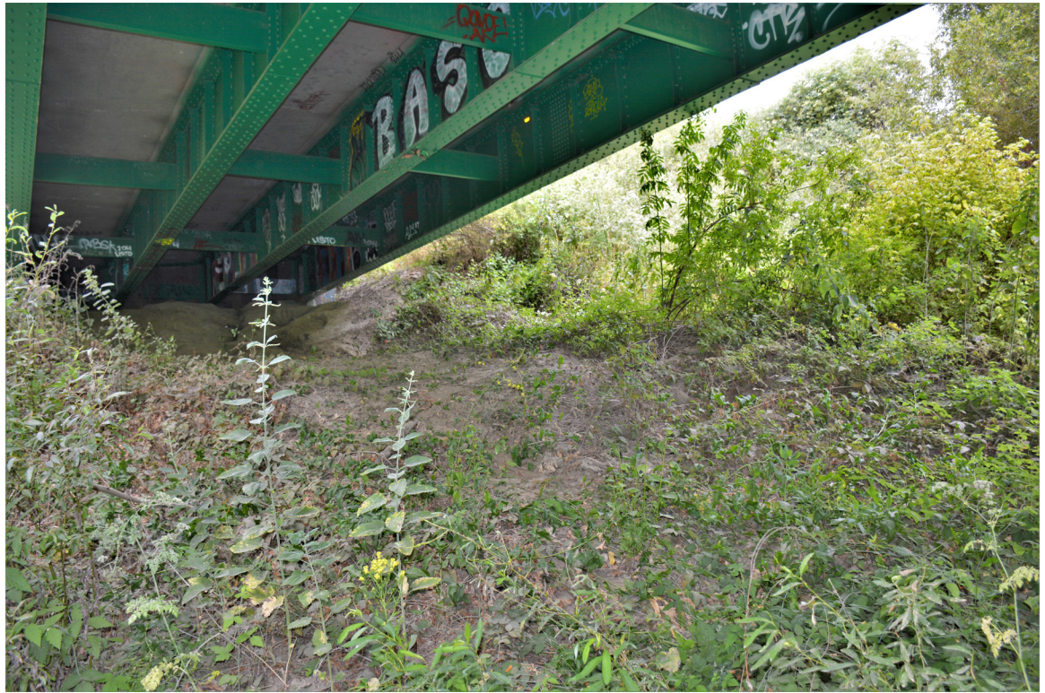
SR 129 Site 5 Pajaro River Bridge. Western section. Photo faces west.
