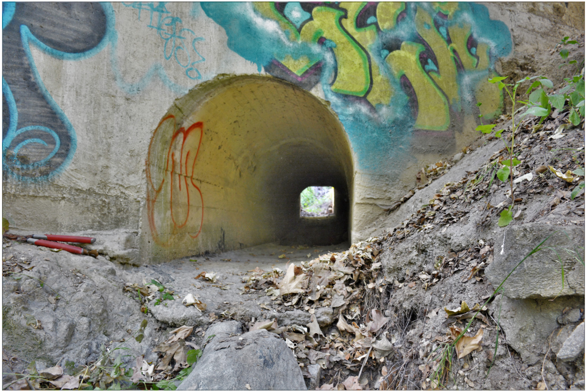
SR 129 Site 8. Southeast arch opening. Photo faces northwest.
