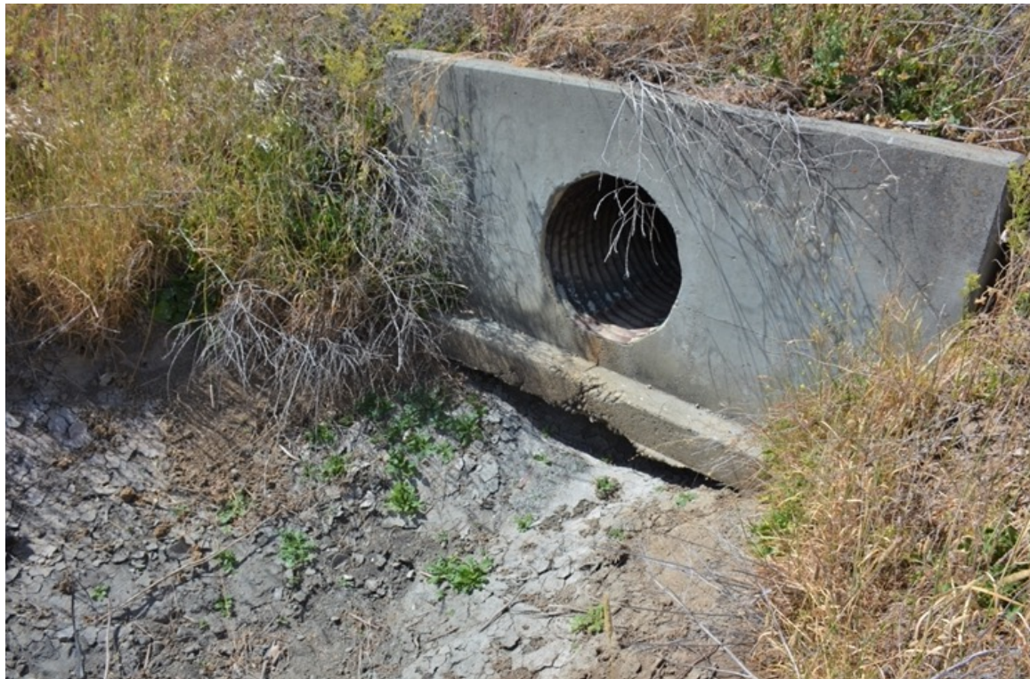
SR 156 Site 4. Southern opening showing raised entrance and concrete ledge. Photo faces northwest.
