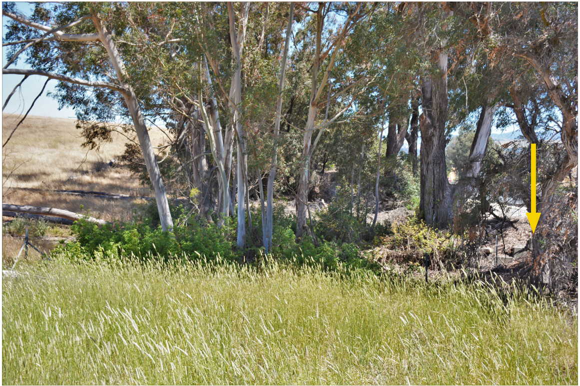
SR 156 Site 1. Another view of the adjacent habitat outside northeastern opening Photo faces east; the culvert opening is indicated by yellow arrow.
