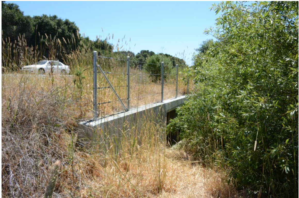
US 101 Site 17. Northern opening with thick vegetation.
