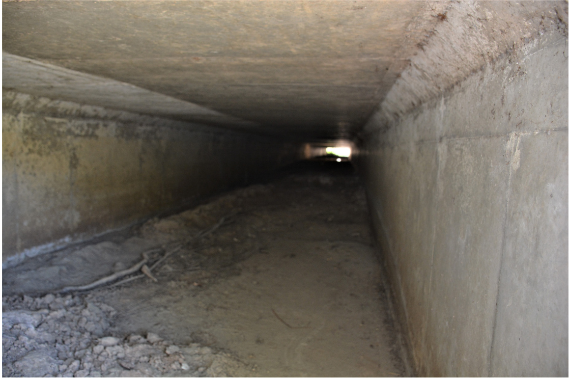
SR 156 Site 5. Inside western culvert, facing northeast to the southwestern opening.
