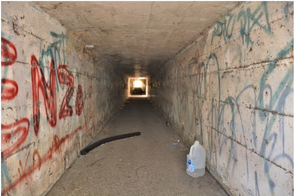
US 101 Site 8. Southern opening close-up. Photo faces north.
