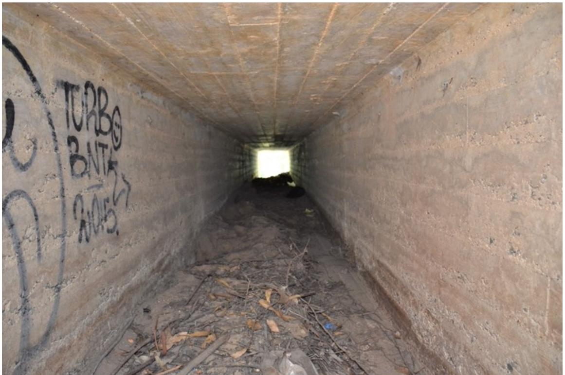
US 101 Site 11. Close-up view facing southern opening.
