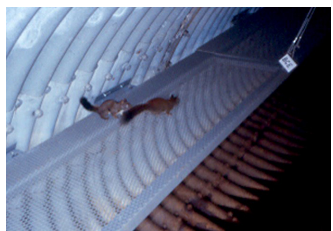
Metal shelving such as the units made by Critter-Crossing allow animals passage through flooded culverts and undercrossings. At top, Professor Kerry Foresman of Critter-Crossing Technology in Montana; middle photos show shelving in a 1.2m wide culvert; lower camera trap photos show small- and medium-sized mammals using the shelving during flooding. Photos courtesy Kerry Foresman.
