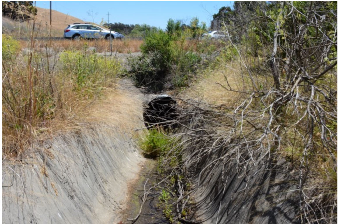
US 101 Site 5. Northwestern opening and concrete levee.
