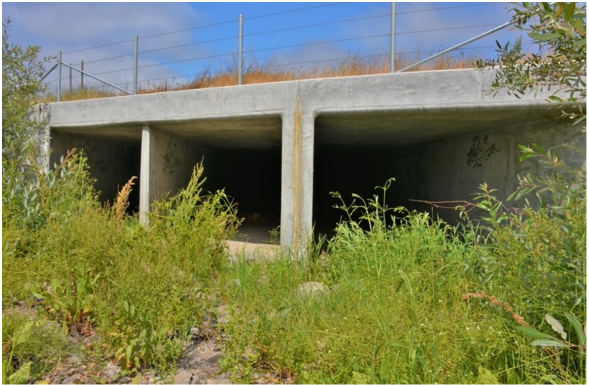
US 101 Site 19. Southeastern opening of triple box culvert.
