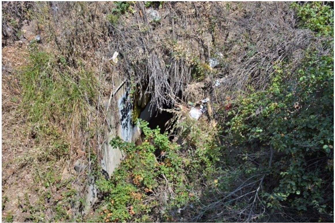
US 101 Site 14. Southern opening.
