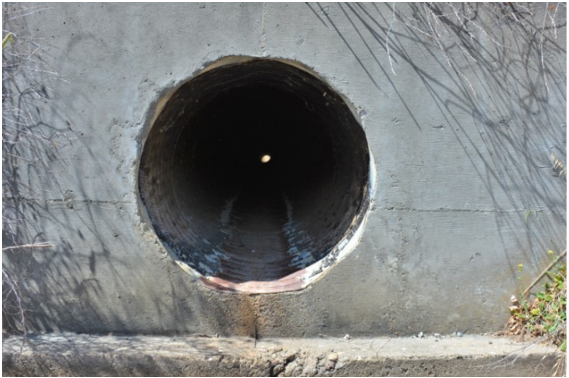
SR 156 Site 4. Close-up of southern opening.
