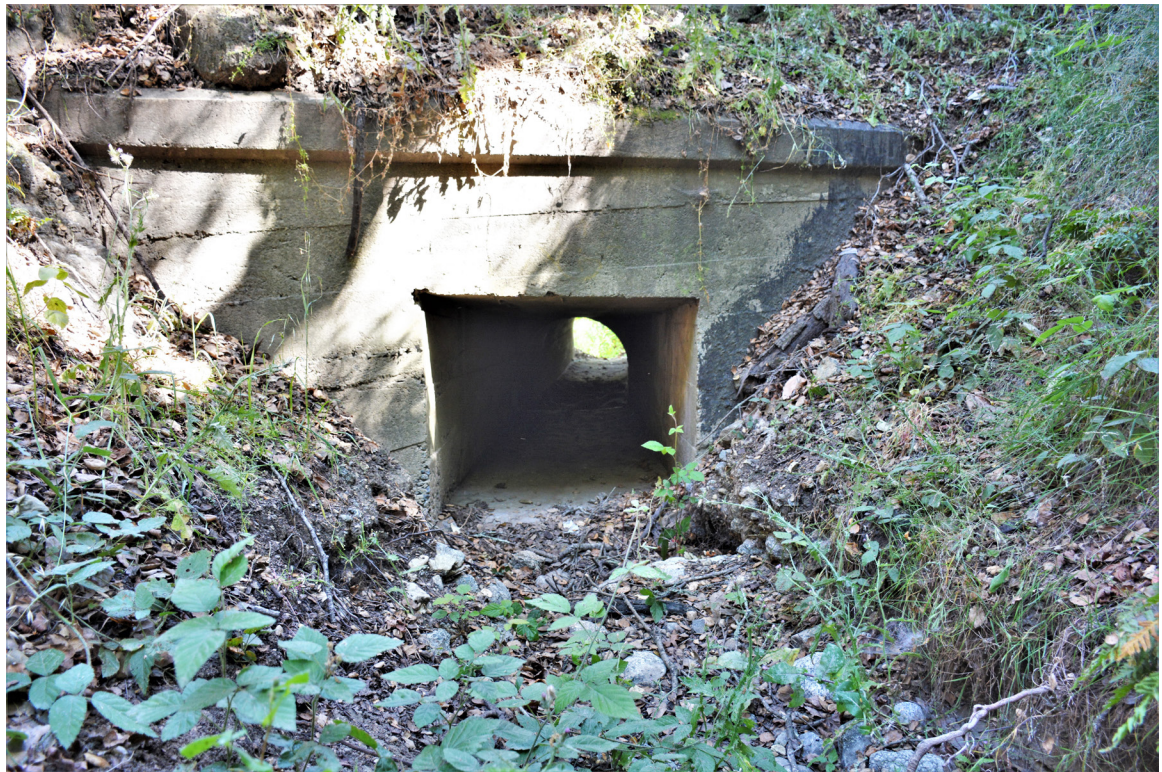
SR 129 Site 8. Northwest square/box opening. Photo faces southeast.
