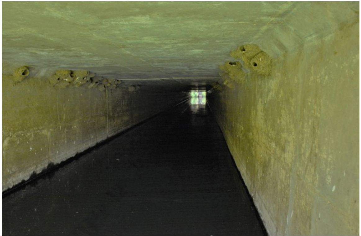
US 101 Site 1. Center section facing northeast.
