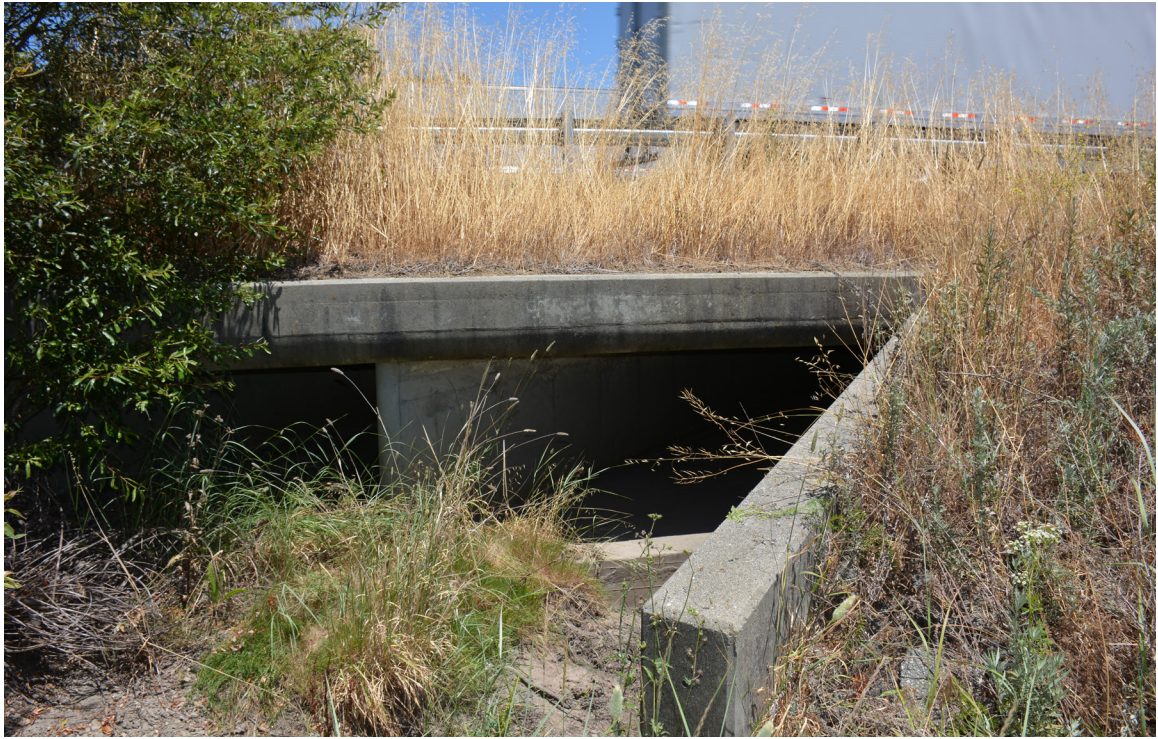
SR 156 Site 5. Southwestern opening. Photo faces north.
