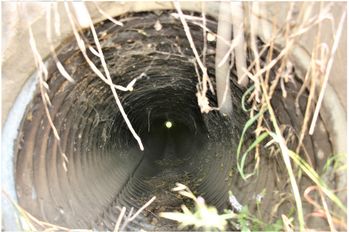
SR 129 Site 1. Close-up of southwest opening. Photo faces northeast.
