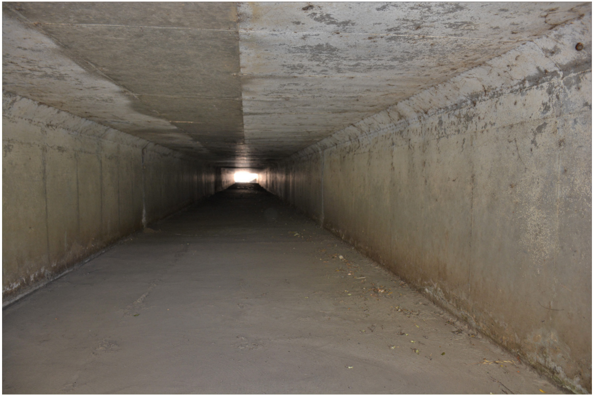
SR 156 Site 5. Inside eastern culvert, facing northeast to the southwestern opening.
