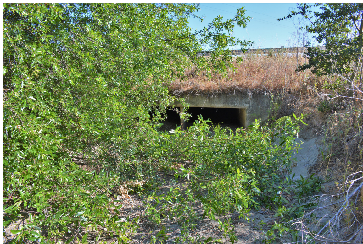
SR 156 Site 6. Northern opening. Photo faces south.
