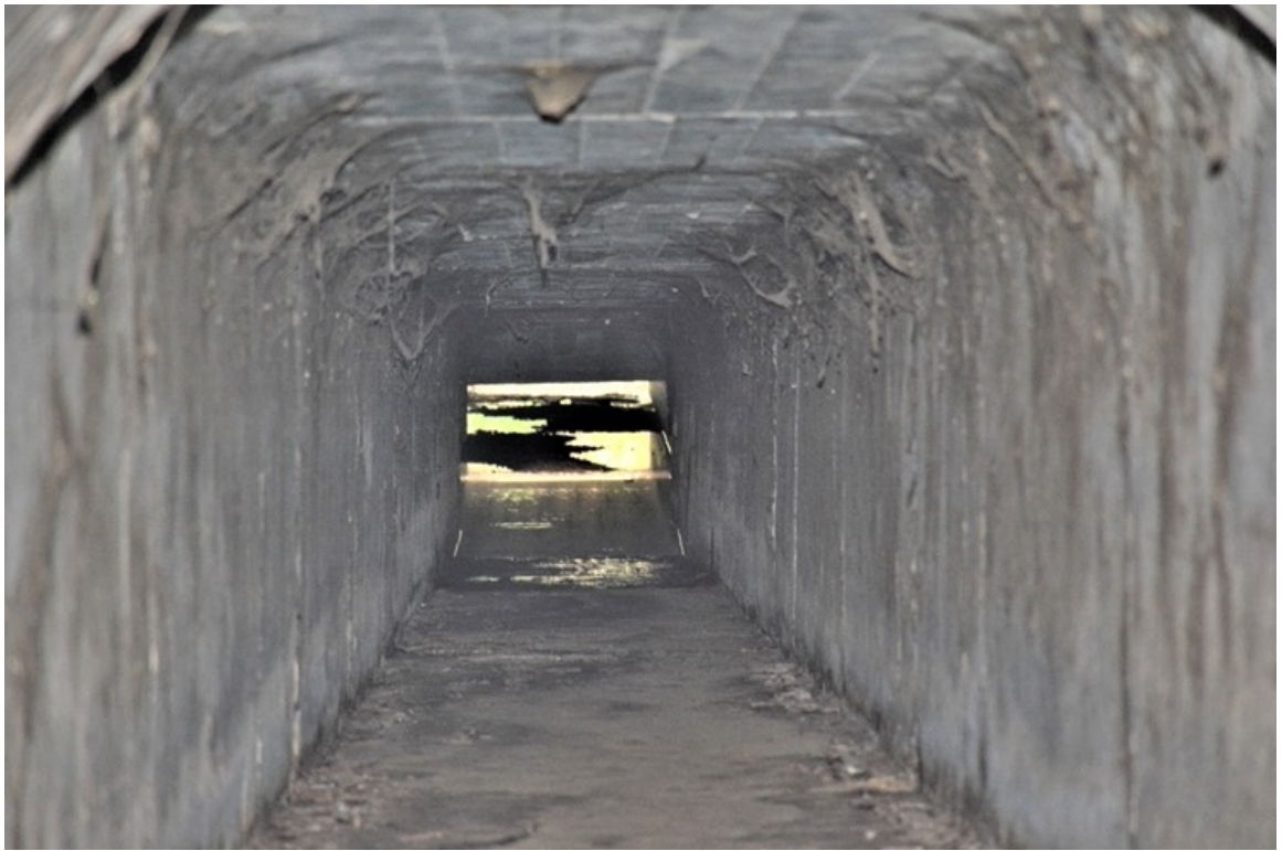
US 101 Site 7. Photo faces the southern opening.
