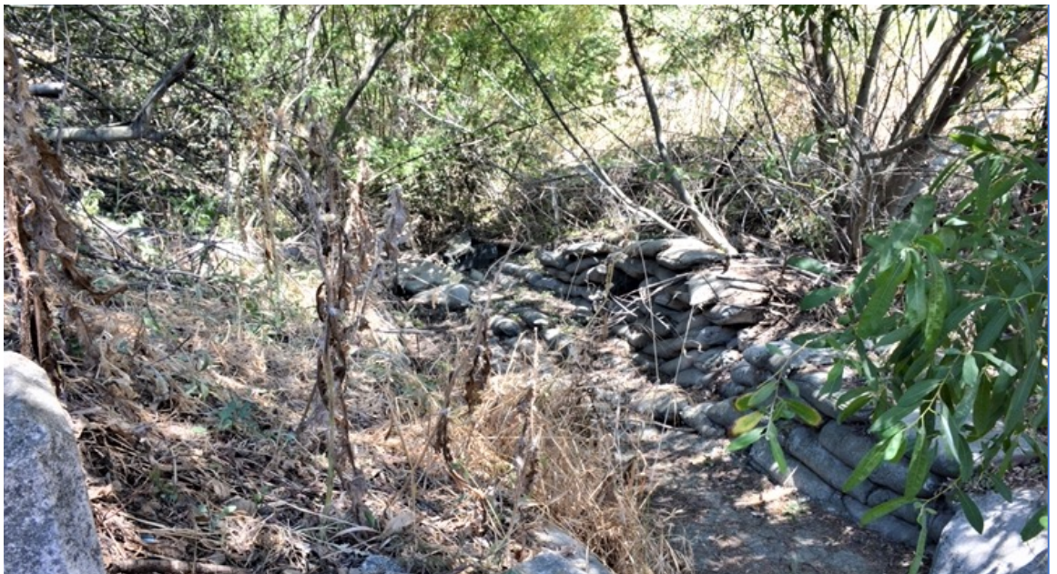
US 101 Site 8. Example of the levee leading to the east.
