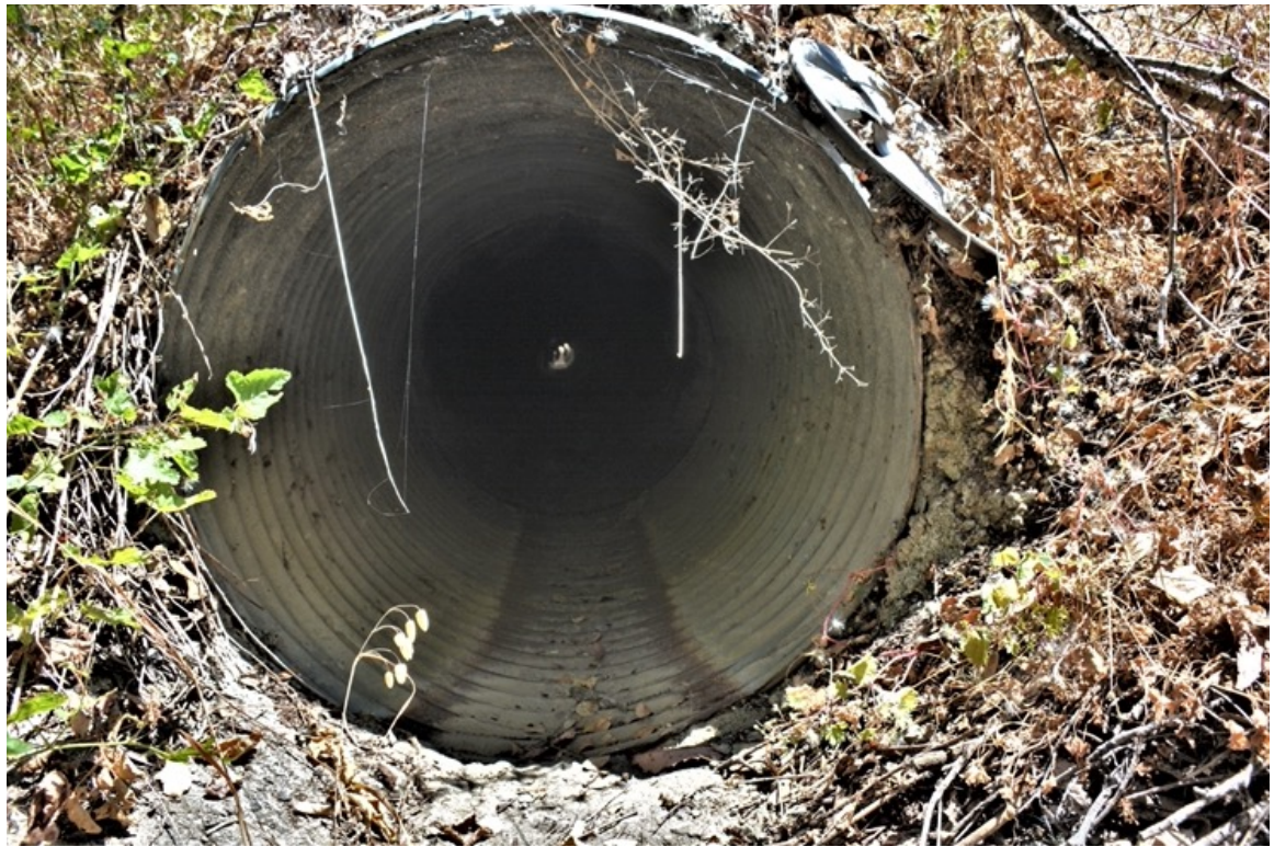
US 101 Site 13. Southern opening.
