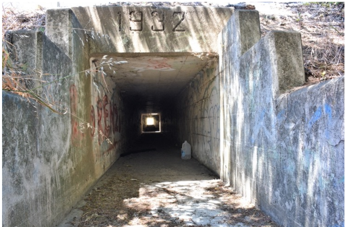
US 101 Site 8. Southern opening.
