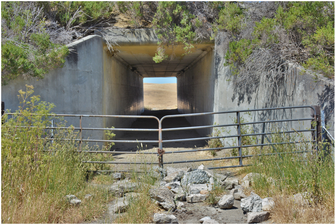
SR 156 Site 3. Southwestern opening with gate in front of entrance.
