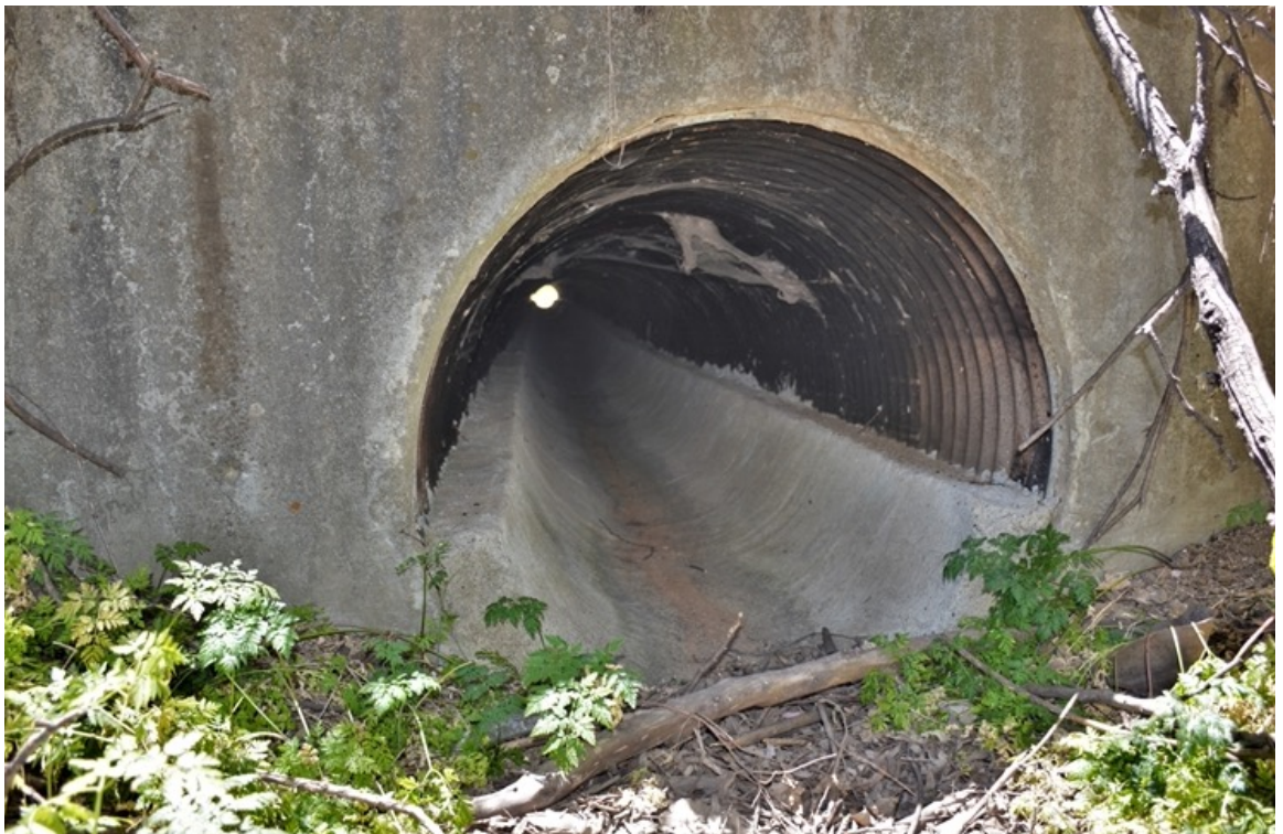
SR 156 Site 2. Close-up of northern opening showing cement bottom.
