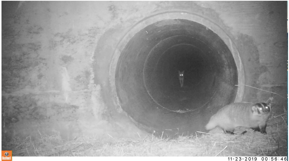
American badger and coyote traveling north through the culvert at SR 152 Site 4 Coyote and badger culvert on November 23, 2019.
