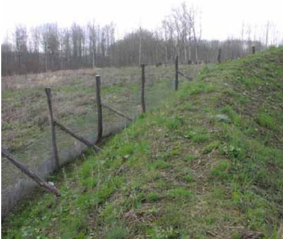
A berm on the side of a wildlife overpass. Photo by Tony Clevenger.
