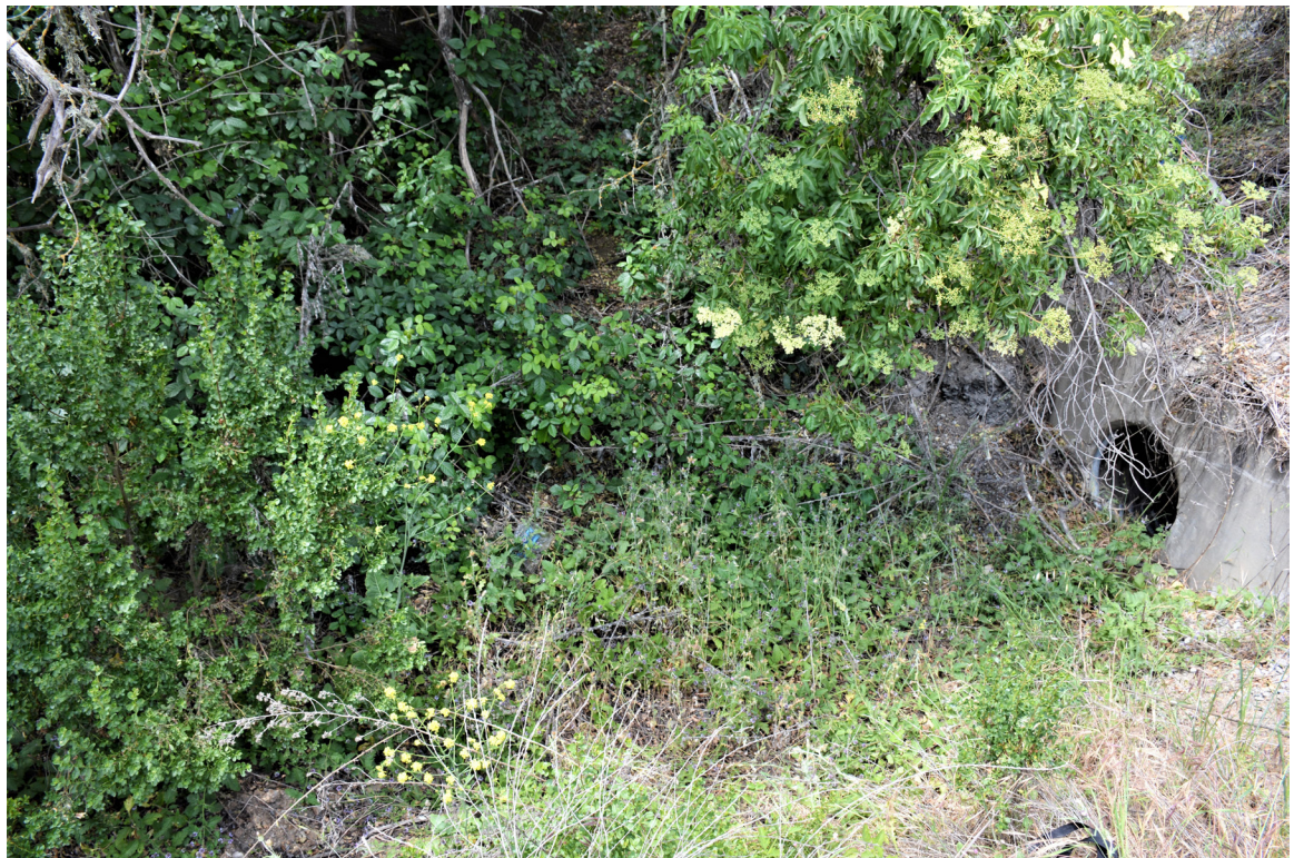
SR 129 Site 1. Southwest opening. Photo faces northwest.
