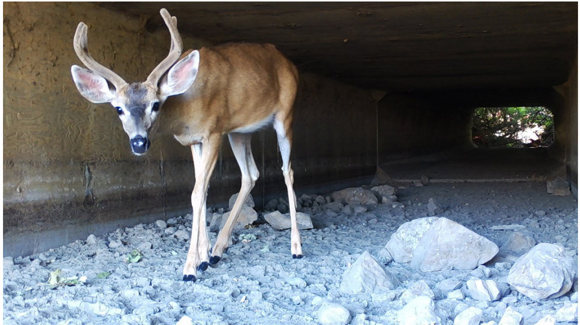
Male deer traveling through the SR 152 Site 2 San Felipe Lake box culvert toward the lake.
