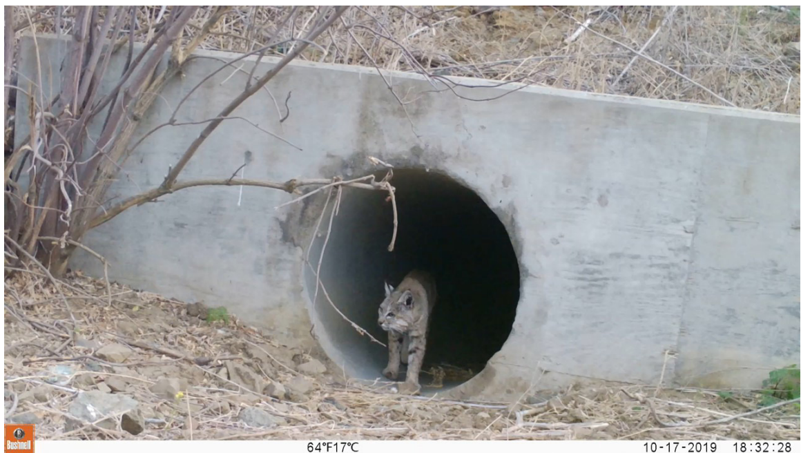
Bobcat traveling through SR 152 Site 6 Tree round culvert
