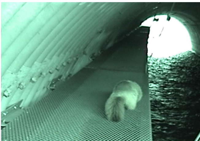
Metal shelving such as the units made by Critter-Crossing allow animals passage through flooded culverts and undercrossings. At top, Professor Kerry Foresman of Critter-Crossing Technology in Montana; middle photos show shelving in a 1.2m wide culvert; lower camera trap photos show small- and medium-sized mammals using the shelving during flooding. Photos courtesy Kerry Foresman.
