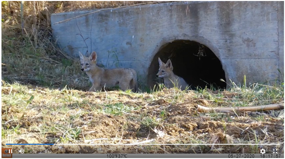
Coyote pups traveling through SR 152 Site 5 Coyote puppy culvert.
