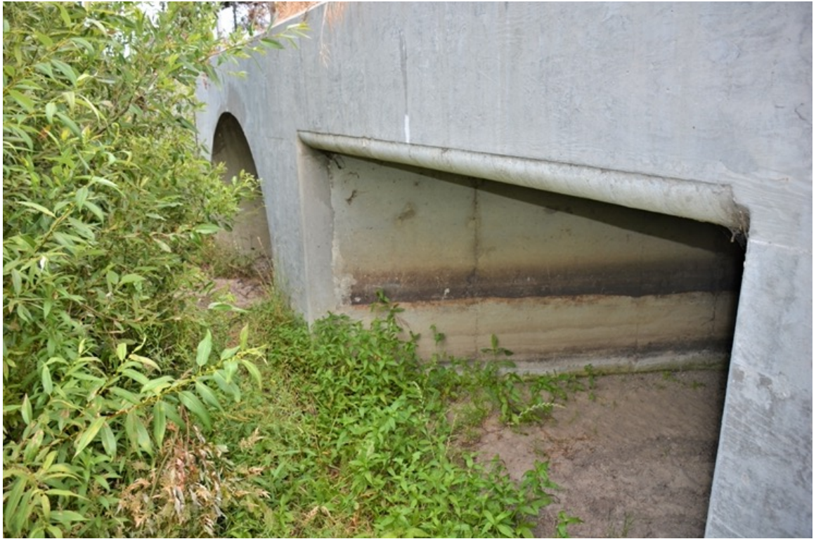
US 101 Site 20A. Northwestern opening of both sections.
