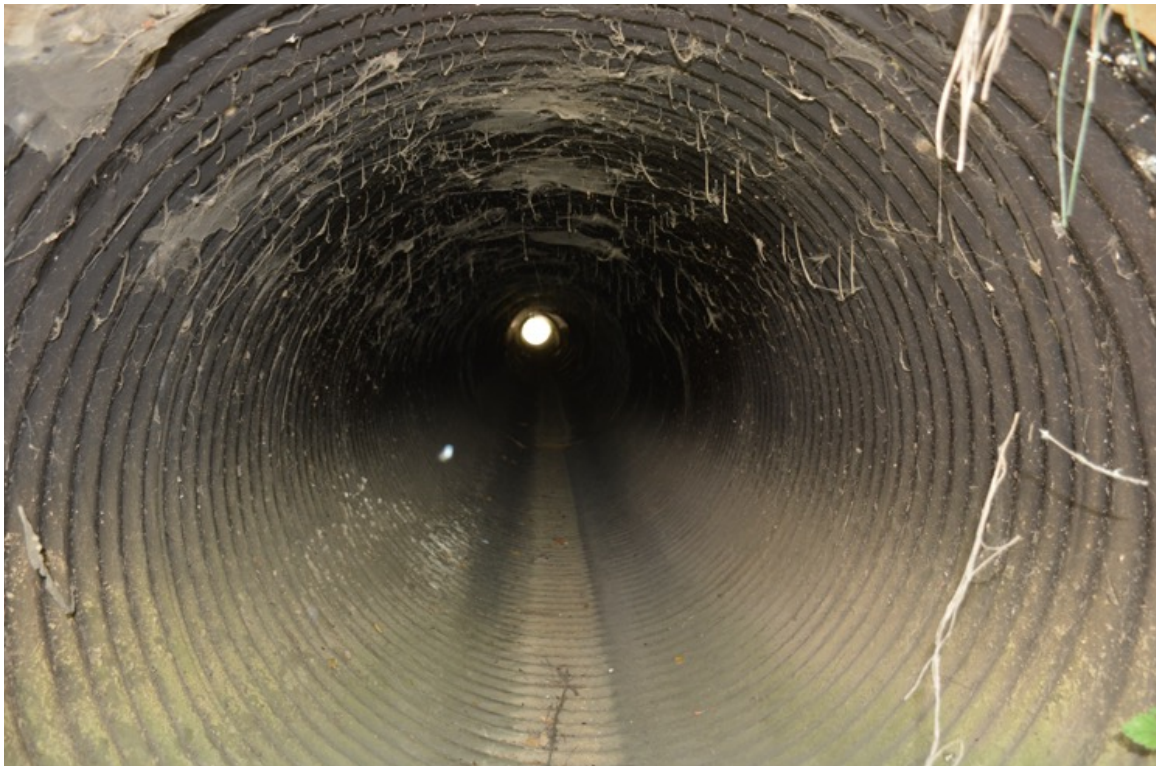
US 101 Site 15. Northern opening close-up.
